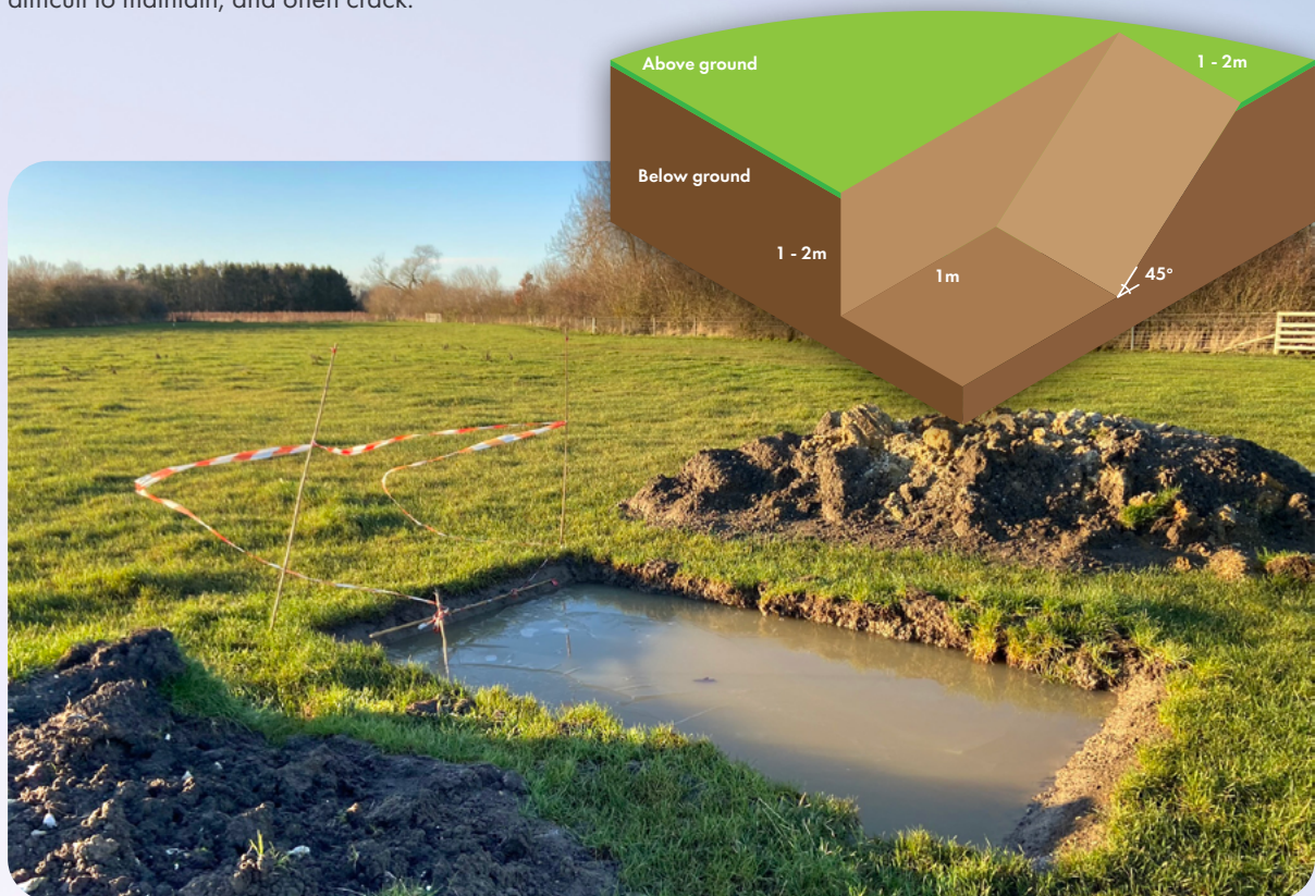
Trial holes are used to assess a new pond's substrate and hydrology before construction begins. © Freshwater Habitats Trust
